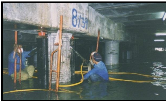
4) WHARF REPAIR, PENANG PORT, MALAYSIA
